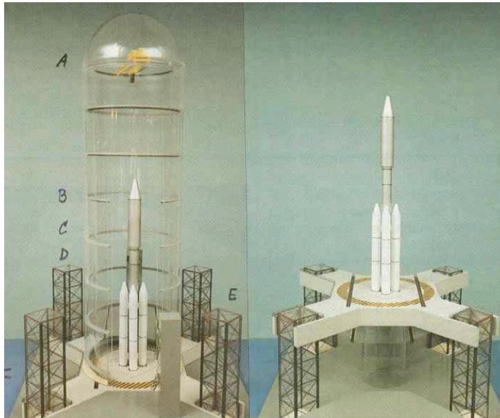
Universal space launch assembly building (B) designed by Brown & Root shown in the model features a polar crane (A), payload environmental cover (C), access door (D), mobile access towers (E) and launch pad jack-up towers (F).
